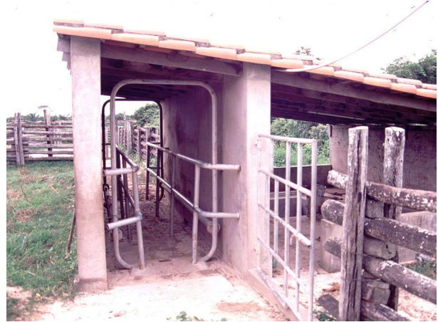
Construction of a spray race. The two spray hoops and connecting pipes, and protective crush bars are shown. The pump and acaricide reservoir are in the section at the right.
